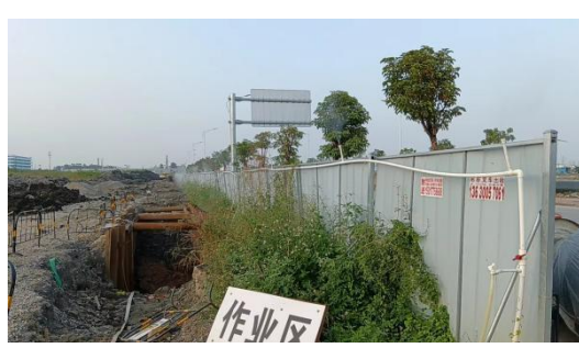
施工围挡及喷淋
